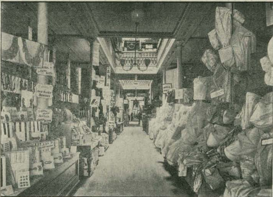
A VIEW OF THE INTERIOR OF THE D.I.C. CASHEL STREET ENTRANCE.—Depth 340 feet.
