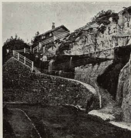
View 11 Entrance to Lot 11 from Clifton Road, showing Cottage No. 3.
