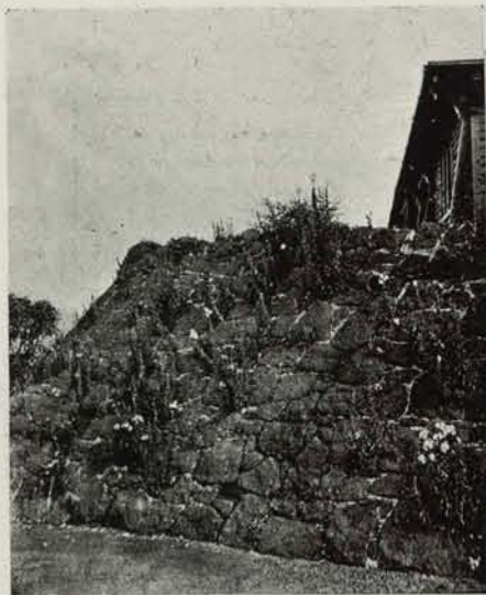
View 7 Red Stone Terrace wall of Cottage No. 1.
