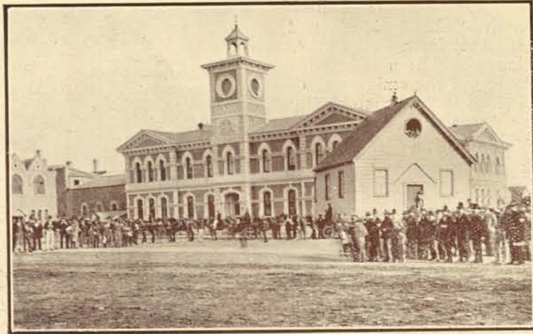
Old Church in course of removal from Hereford Street to Oxford Terrace.
