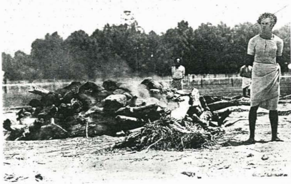
HEATING THE OVEN.
